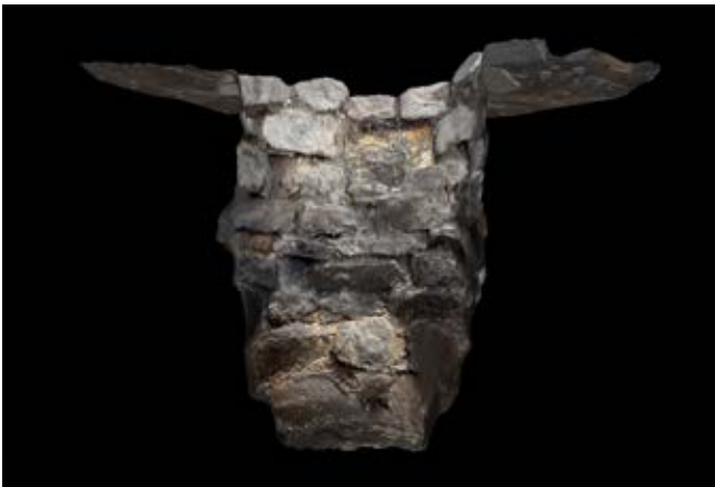
Figure 8: Profile of the stone-lined roadside well. Image captured from a 3D scan.
