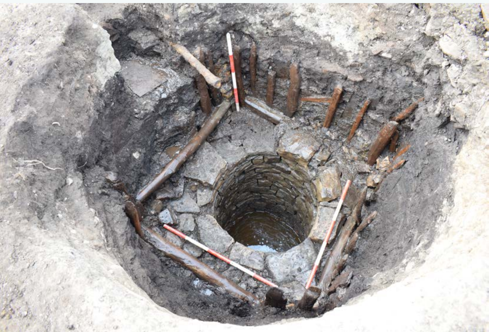
Figure 19: The timber frame used to brace the construction cut for the post-medieval well.
