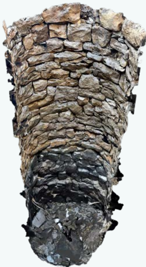
Figure 20: The lower section of the drystone well shaft, post-excavation. Image captured from a 3D scan.
